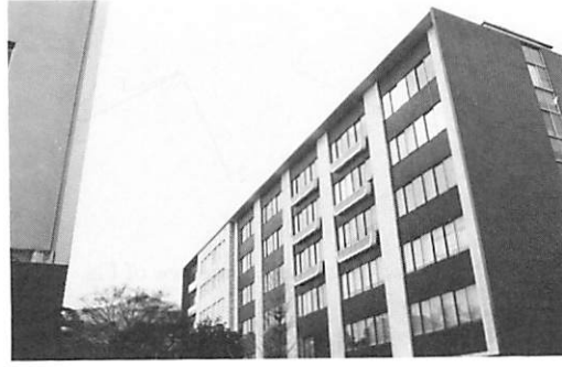
FIG. 7. Image of a building. The upper-right corner has three mutually perpendicular edges.
