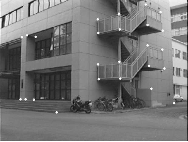
Fig. 7. An image of a real building
